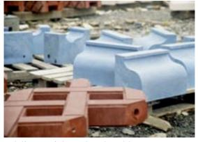
A delivery of through-colour blue 'cyma-reversa' units and through-colour red balcony 'Cancelli' spandrels, waiting to be hoisted into place. I call this material 'photolithic'. It combines the qualities of the pure, ethereal, light (phos) that is chromaticity, with those of dark matter (lithos) which is solid, heavy, mass. The ancient distinction between surface and body, appearance and reality, is now, by this technology, abolished.
